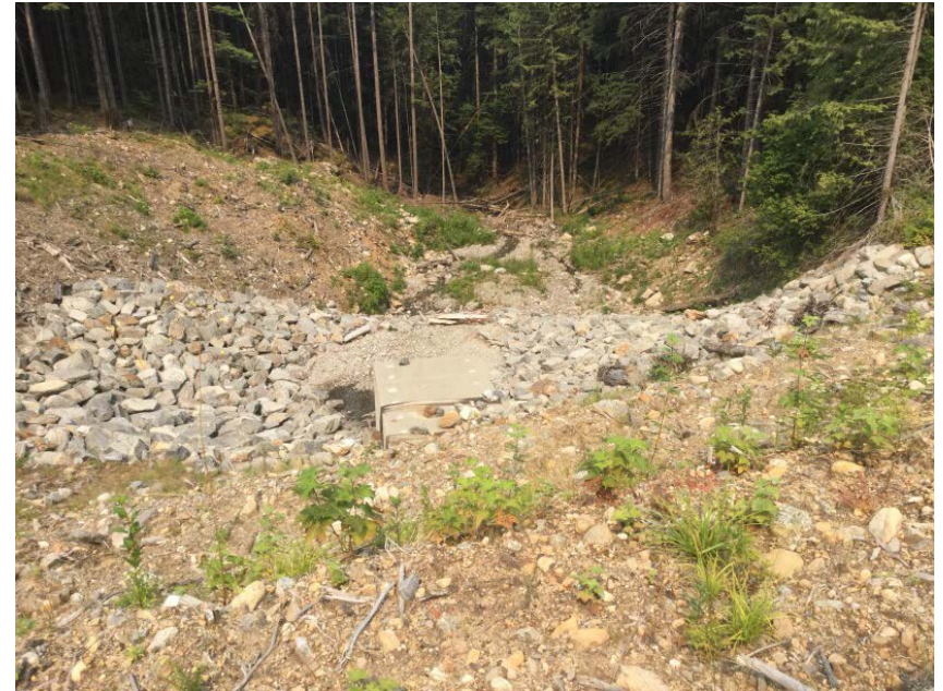
Looking downstream from road surface
