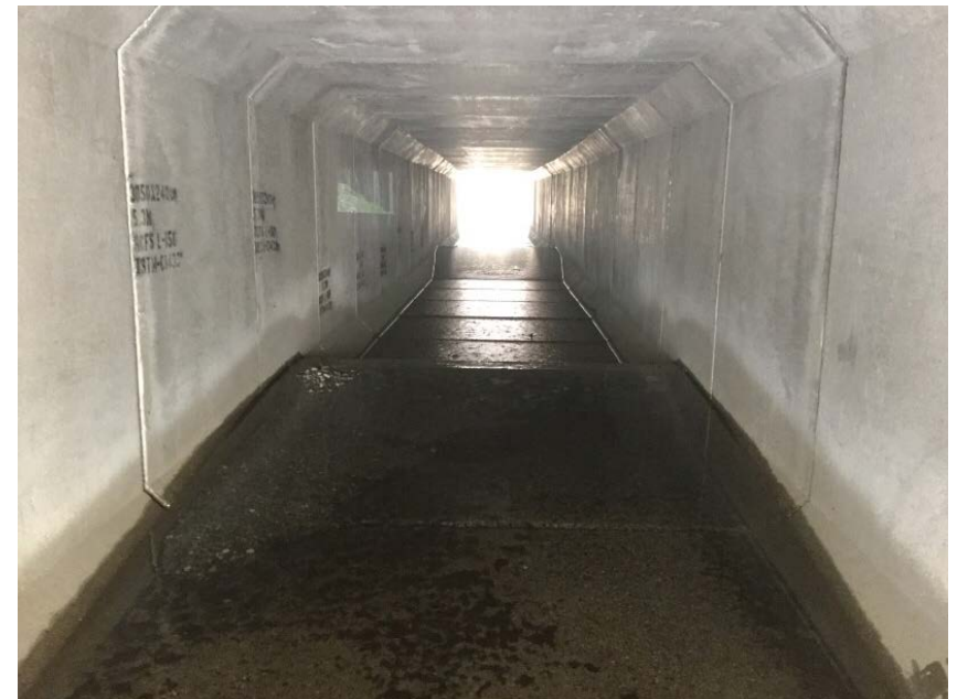
Looking through culvert from inlet
